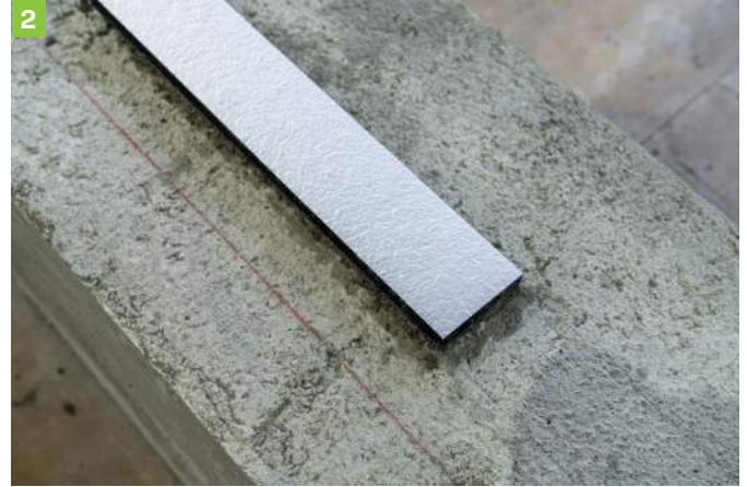
... and place the strip to the concrete bottom beam (silver side upwards).
