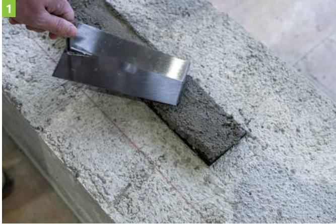
Apply thin layer mortar to the fleece of the middle strip REGUPOL INODIS horizontal ...
