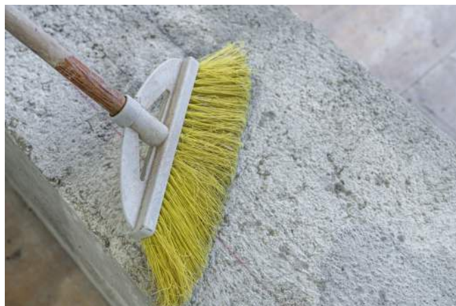
... Clean and free of dust surface.
