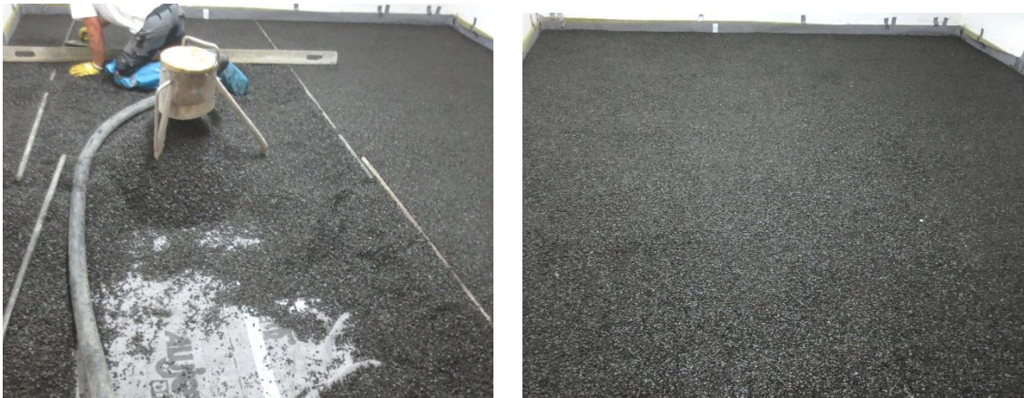
Figure A 2.2: situation during mounting - installation of floor compensating and sound insulating fill
