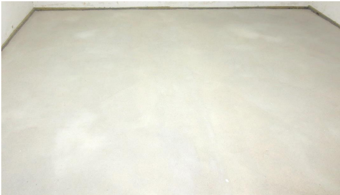
Figure A 2.5: cement screed (situation of test)
