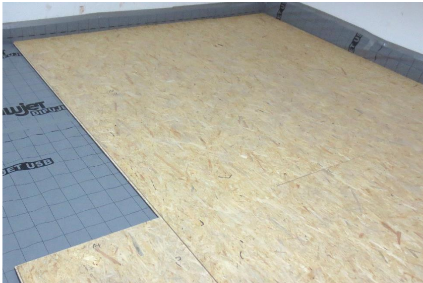
Figure A 2.4: situation during mounting - dry screed
