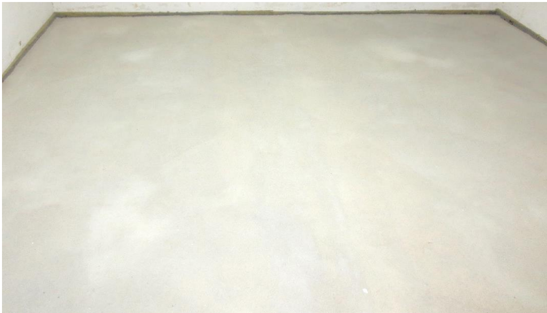
Figure A 2.5: cement screed (situation of test)
